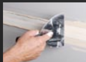
Bed tape in with joint knife or taping knife
